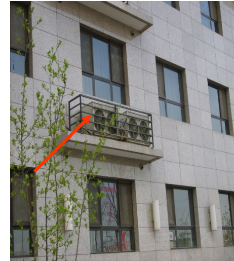
D. 26 floors, 2004, 132m 2 one outdoor & multi indoor units
