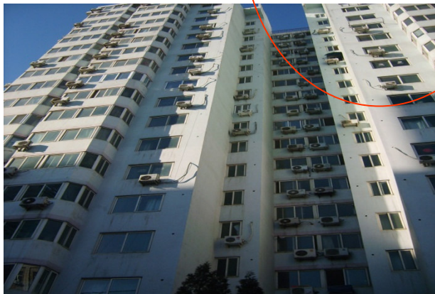
B. 18 floors, 1996, 103m 2 /unit, Split unit
